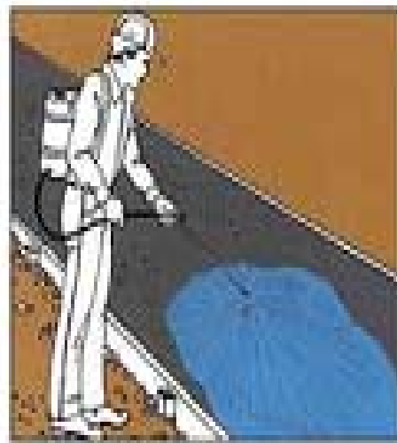
Chemical or liquid membranes reduce evaporation by sealing the concrete.
