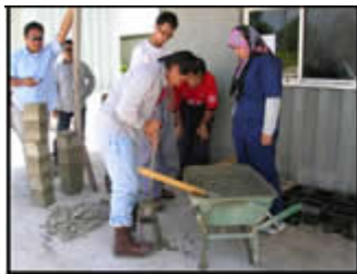
Concrete Slump Test
