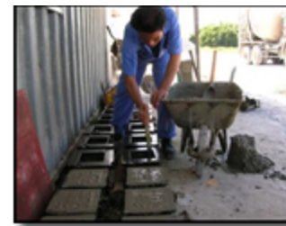
Concrete Cube Preparation
